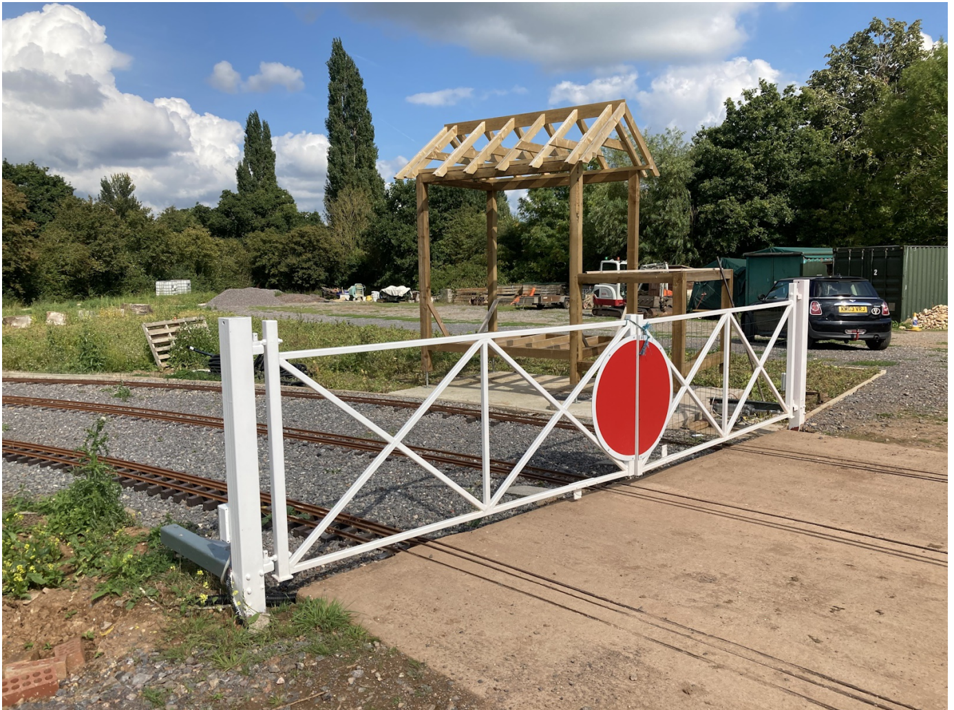
Fig 7 - Signal Box - Under Construction
